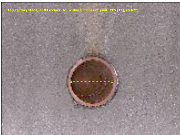
Photo: 7_8A, Media No.: 010208_1 186.42FT, Tap Factory Made, at 03 o'clock, 6", within 8 inches of joint: YES
