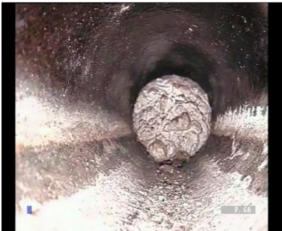
Photo: 4_6A, VCR No.: 010208_1 30FT, Obstacles Other, 100 %of cross sectional area, from 12 to 12 o'clock
