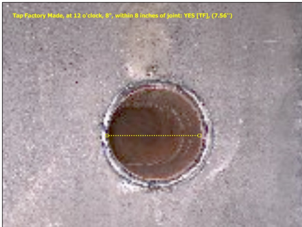
Photo: 7_9A, Media No.: 010208_1 238.89FT, Tap Factory Made, at 12 o'clock, 8", within 8 inches of joint: YES
