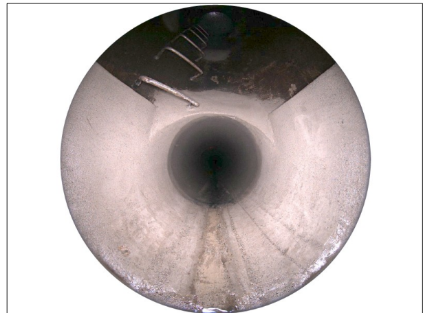
Photo: 7_11B, Media No.: 010208_1 262.8FT, Downstream Manhole, Survey Ends / END
