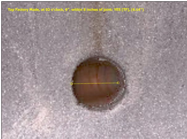
Photo: 7_7A, Media No.: 010208_1 177.99FT, Tap Factory Made, at 02 o'clock, 6", within 8 inches of joint: YES
