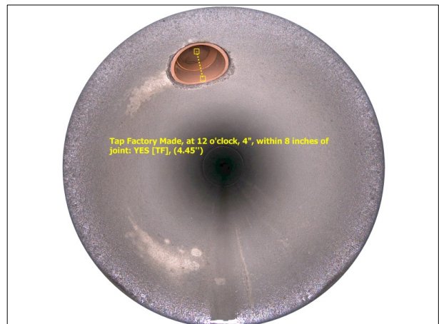
Photo: 7_6B, Media No.: 010208_1 136.98FT, Tap Factory Made, at 12 o'clock, 4", within 8 inches of joint: YES
