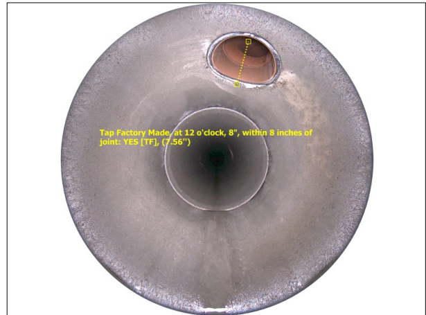
Photo: 7_9B, Media No.: 010208_1 238.89FT, Tap Factory Made, at 12 o'clock, 8", within 8 inches of joint: YES
